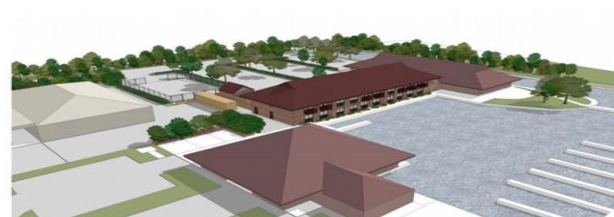
Aerial View North East
