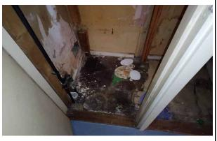
Asbestos was identified in both the vinyl floor tiles and the bitumen adhesive. Any material underneath asbestos containing bitumen adhesive must be presumed to contain asbestos as the materials will not be able to be separated from the adhesive.
