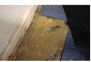
Any material overlaying or underneath asbestos containing bitumen adhesive must be presumed to contain asbestos as the materials will not be able to be separated from the adhesive.
