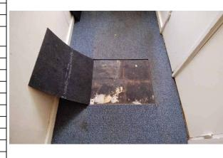
Any material overlaying or underneath asbestos containing bitumen adhesive must be presumed to contain asbestos as the materials will not be able to be separated from the adhesive.
