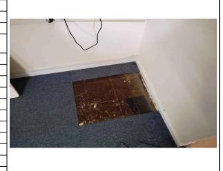
Asbestos was identified in both the vinyl floor tiles and the bitumen adhesive. Any material underneath asbestos containing bitumen adhesive must be presumed to contain asbestos as the materials will not be able to be separated from the adhesive., Tile and Bitumen
